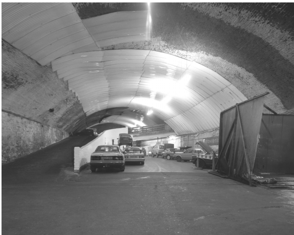
The site of the former Dingle Station on the Liverpool Overhead Railway - now a car repair workshop Photo Nick Catford
